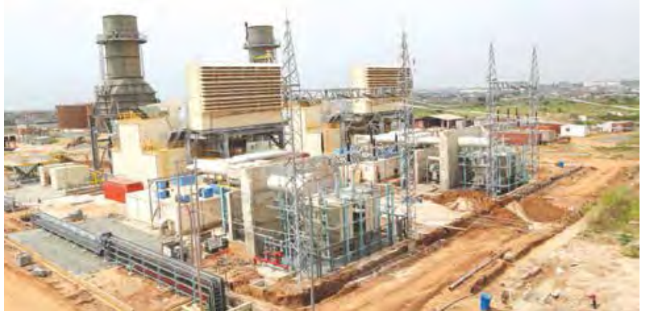
An Aerial view of the Kpone Thermal Power Plant
