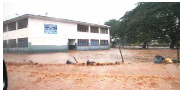
Kyease Cluster of Schools compound submerged in water
