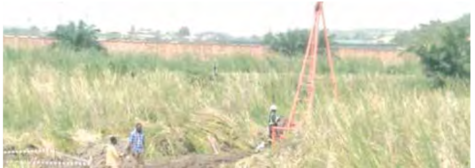
Geotechnical investigation in progress at the selected Site in January 2015
