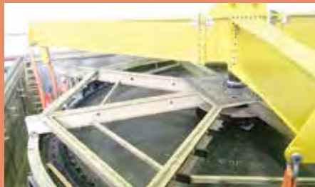
Jig fixed to the upper bracket of stator frame.
