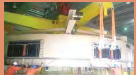
Stator being guided to rest safely on metal supports at the erection bay
