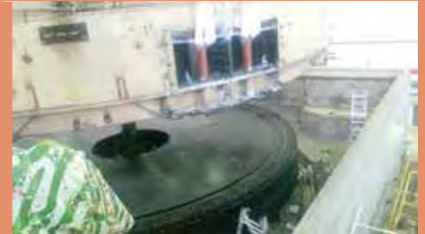
Stator frame gradually being lifted
